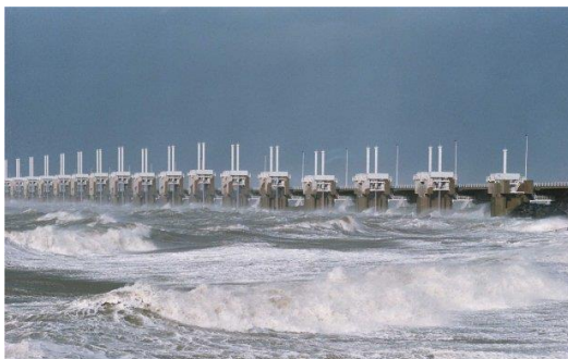
Storm Surge Barrier Oosterschelde
