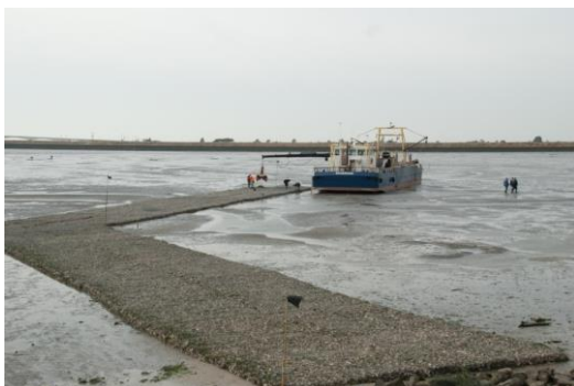
Oyster reef construction Oosterschelde
